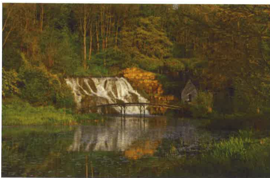
Reservoir Act compliance works to Blenheim Dam – cost £1.5m
